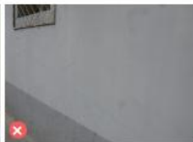
墙体采用抹灰涂料覆盖
