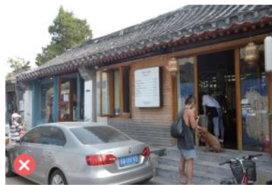
外立面装修、装饰中私自改变建筑外观 ▶
